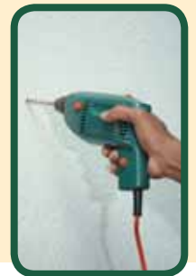
Wall plug Installation
